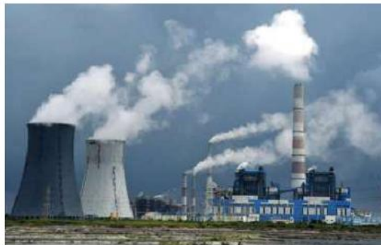
Thermal boost: The capacity of the Thoothukudi Thermal Power Station will be increased. It will have a total installed capacity of 1,600 MW as against the present 1,050 MW. FILE PHOTO
